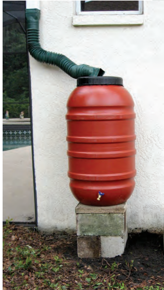
Place the barrel on top of blocks and place the gutter attachment on top of barrel opening.
