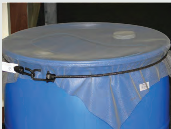
Screen placed over the barrel opening will keep leaves and other debris out of the barrel. For screw top barrels (left), the screen can be held in place with the screw top lid. For other barrel types (right), the screen can be held in place with a rope or stretch cord.
