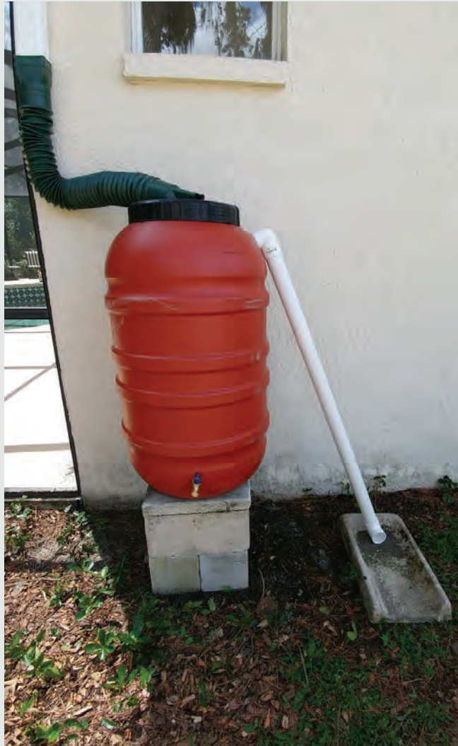
Direct the overflow pipe away from the house foundation. This is a completed installation for one rain barrel.
