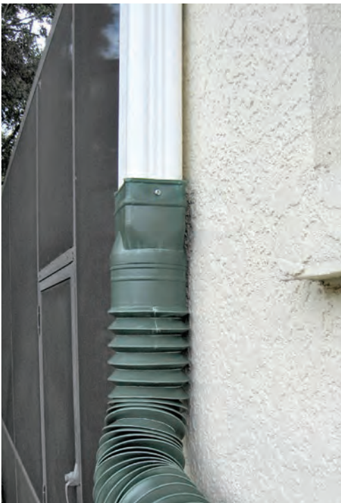
Based on the height of barrel, mark and cut the downspout, then securely attach the pipe or flexible downspout attachment with sheet metal screws or rivets.
