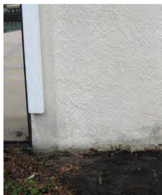
Ground should be level and clear of debris.
