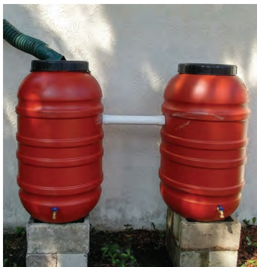
Attach two-inch PVC pipe to connect the barrels.
