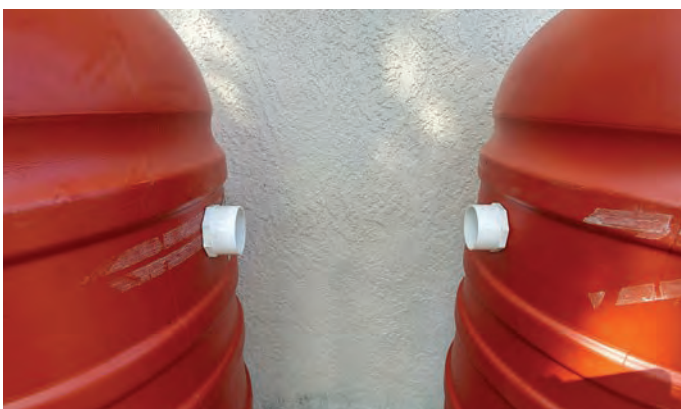
Place two-inch PVC male adapters in each barrel.
