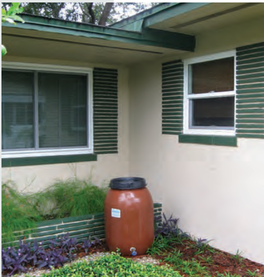
Rainwater shedding off this roof can still be captured, even without gutters.
