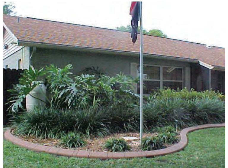
The large surface area of this roof provides a great catchment area for rainwater. Notice how the rain barrel blends into the landscape.
