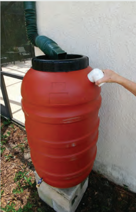
Direct the overflow pipe away from the house foundation. This is a completed installation for one rain barrel.
