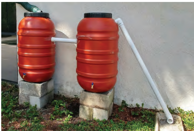
Place an overflow outlet on the second barrel (or last barrel if multiple barrels are connected together). Installation is complete.
