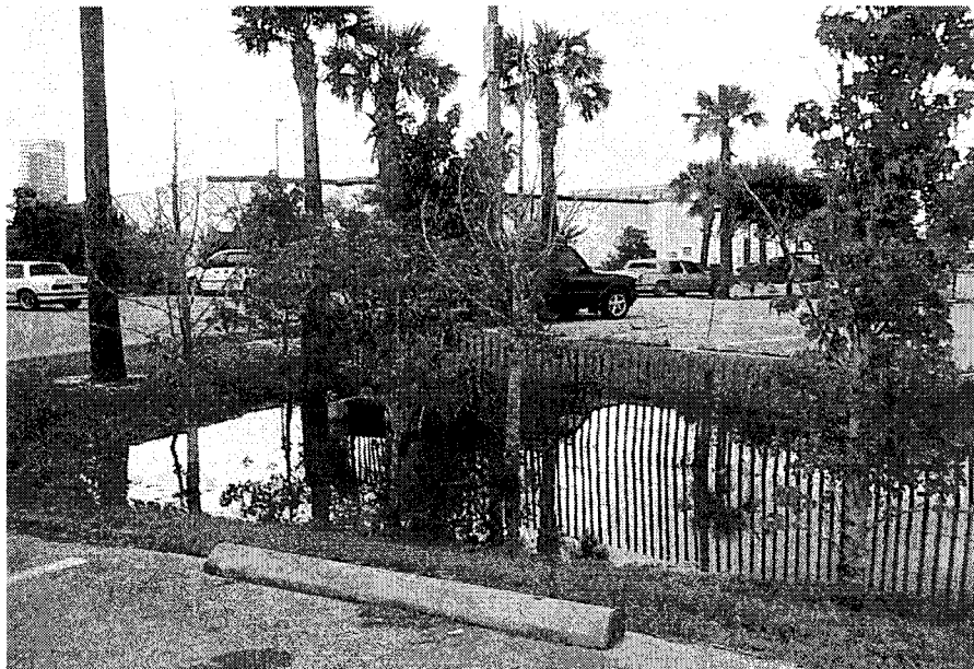
POROUS PAVEMENT WITH PLANTED SWALE IN POOR CONDITIONS BECAUSE PEOPLE HAVE REMOVED THE FENCE AND TAKEN SHORT CUTS ACROSS THE SWALE
