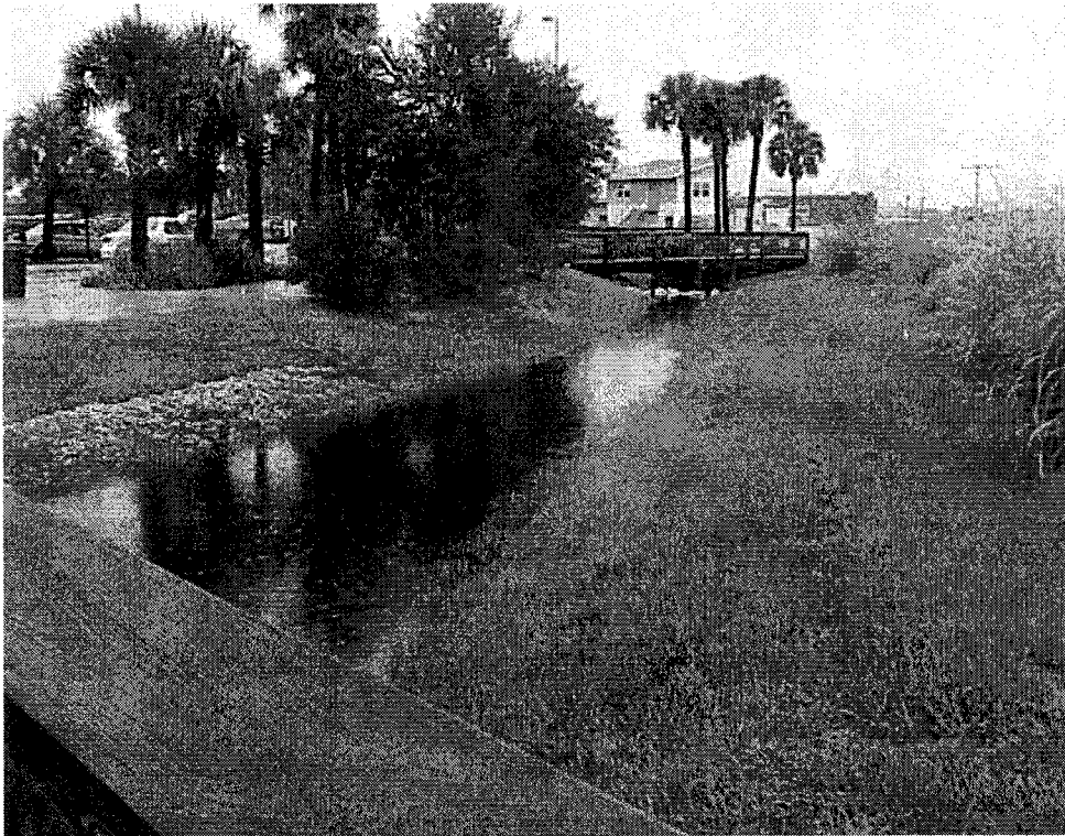
THE STRAND AFTER THE BERM REPAIRS SHOWING NEW SIDE BANK FILTER
