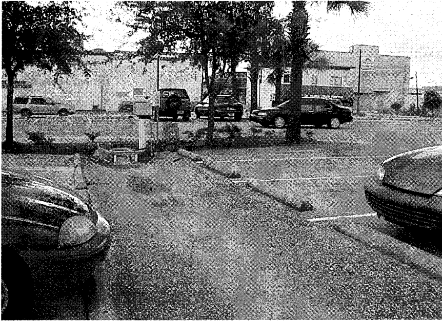
ASPHALT PAVEMENT WITH NO PLANTED SWALE
