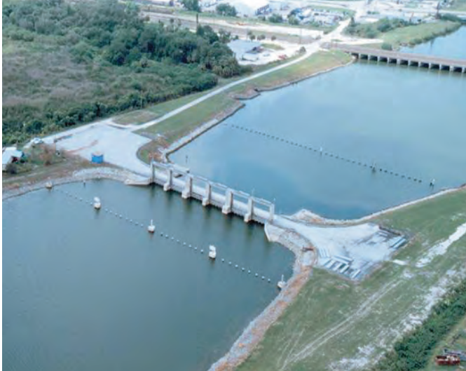
One of the large structures on the Tampa Bypass Canal.
