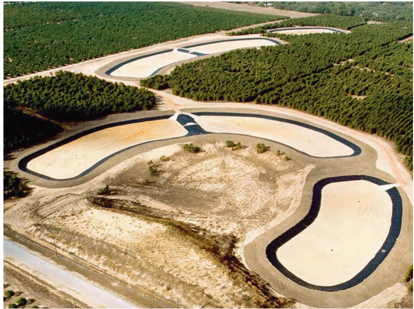
The construction of large rapid infiltration basins (RIBs) for recharging aquifers with large quantities of highly treated reclaimed water is a potential water resource development project for the Tampa Bay Planning Region.
