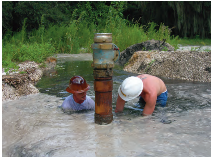
District technicians work to plug an abandoned free-flowing well.
