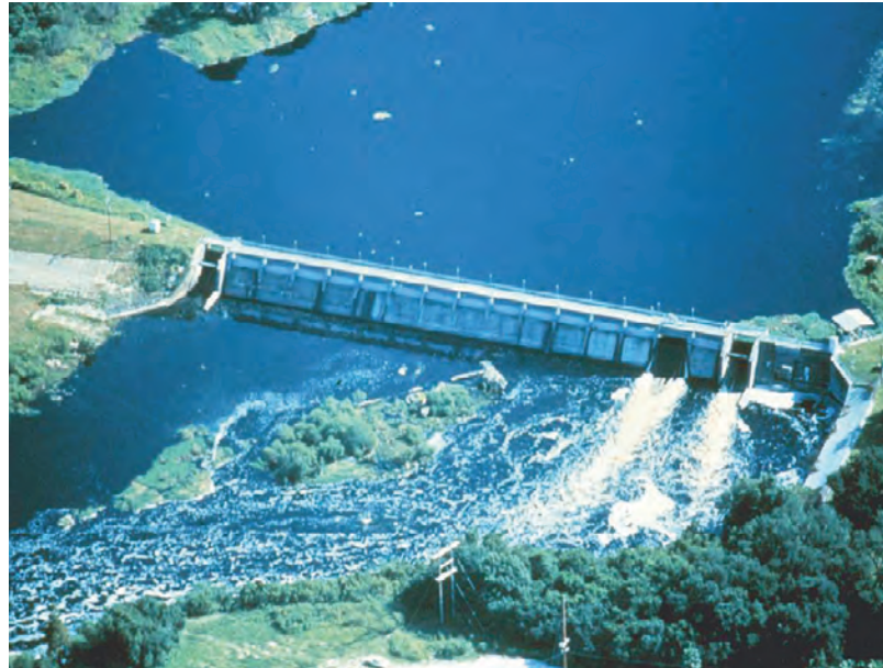
Water flowing from the City of Tampa's dam during a higher-flow period.
