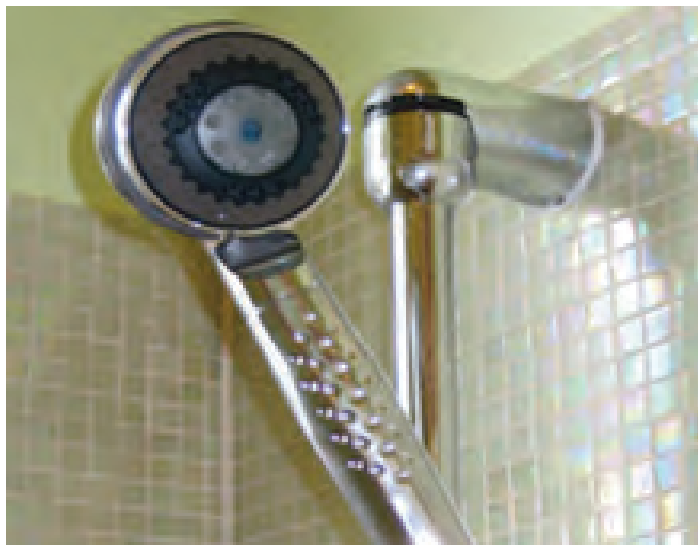
Low-flow showerheads are one of a number of water-conserving fixtures that can significantly reduce indoor water use.
