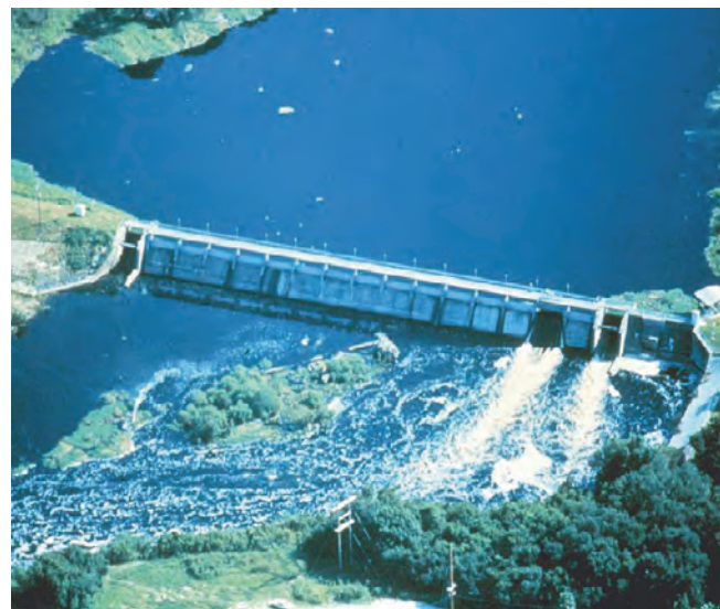
The City of Tampa's dam on the Hillsborough River creates a small reservoir that provides the majority of the city's potable water supply.
