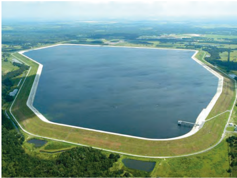
Tampa Bay Water's C. W. Bill Young Regional Reservoir in southern Hillsborough County. The reservoir has a 15-billion-gallon capacity and receives water from the Alafia and Hillsborough rivers and the Tampa Bypass Canal.
