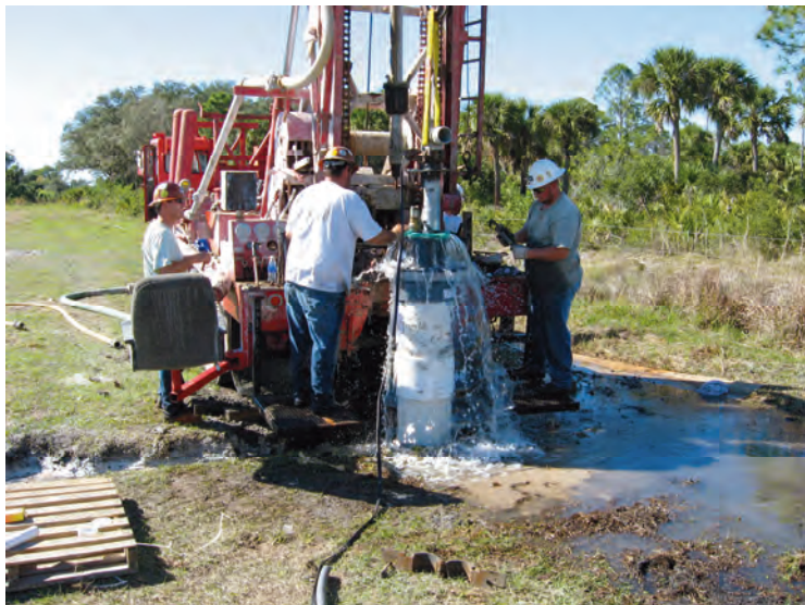
The construction of a groundwater production well.
