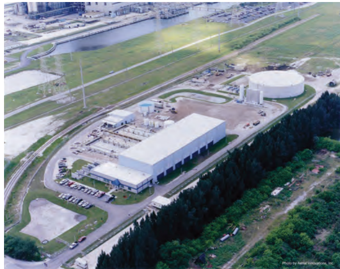
Tampa Bay Water's facility on Tampa Bay is the largest seawater desalination facility currently in operation in North America.
