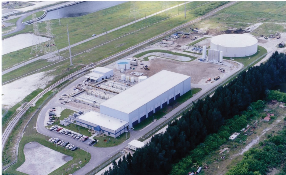
Tampa Bay Water's facility on Tampa Bay is the largest seawater desalination facility currently in operation in North America.
